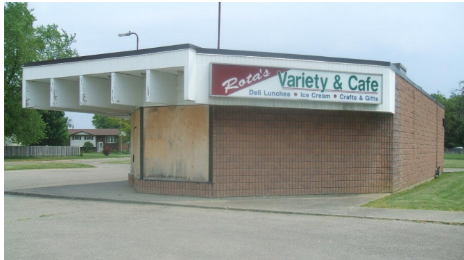
Our new building is located at 850 Wallace Street in Wallaceburg. Ample parking and lighting are just 2 of the great features.
